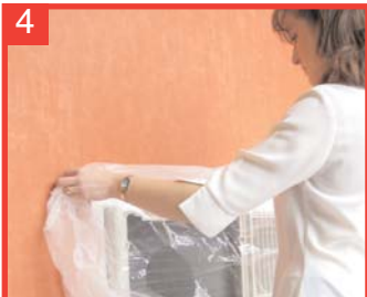
4 Place and fix an AC-OK Cleaning Cover around the unit...
